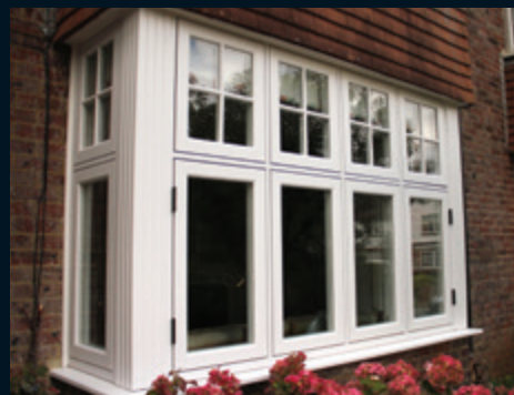
Flush external finishes with equal sightline
