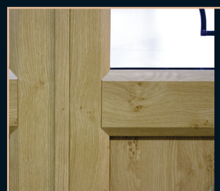
115 mm midrail upgrade
